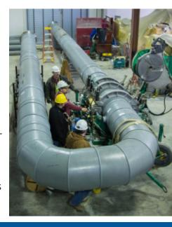
The material is 100% recyclable and environmentally friendly. It also lasts significantly longer than traditional pipe materials because it will not corrode. PP-RCT will outlast the building in which it is installed. "Overall, the idea of thermoplastic pipe for hydronic applications is a sign of the future," said field foreman Scott Rick from Midwestern Mechanical, Inc. in explaining
