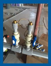
"Heat fusion means no need for joints, glues, or solvents, ultimately leading to a more solid pipe."
