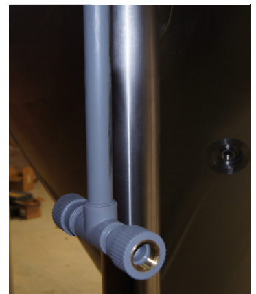
Valve of PP-RCT installed at Birdsong Brewery
