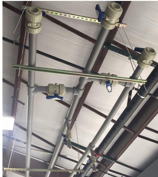
Installation of PP-RCT piping at Compass Rose
