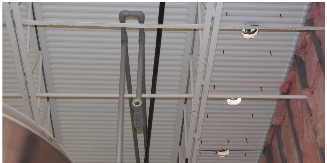
PP-RCT ready to be connected to the vats inside Birdsong Brewery
