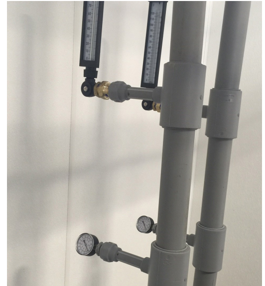
Psi gauges for the set of pipes at Compass Rose
