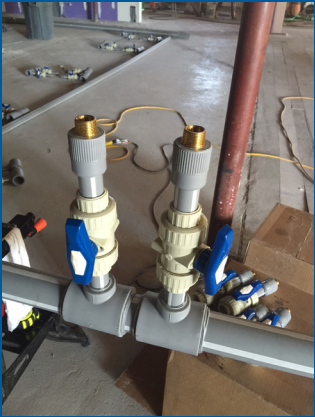
Pipe fused on site at Ponysaurus
