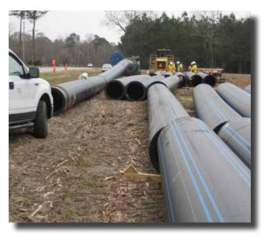
Pipe onsite being fused to ger ready for installation via horzontal directional drilling.
