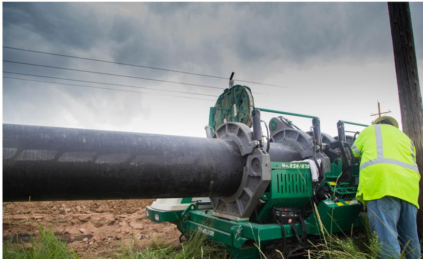
ongoing maintenance expenses.” The corrosive soil and high ground water levels eliminated metallic materials. Ultimately, the fusibility and flexibility of HDPE PE4710 made it the best, most cost effective choice for Victory.
