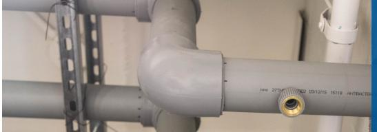
Durable, corrosion-free pipe installed over an operational laboratory.
