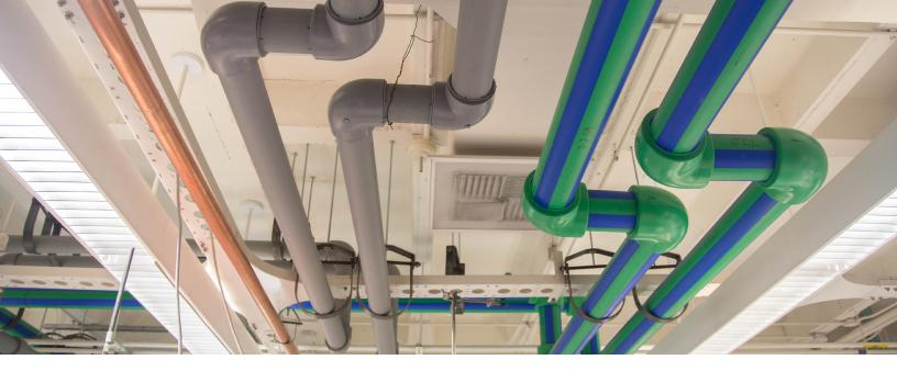
Another product was specified for the chilled water line but was not approved for the hot water return. In the end, PP-RCT, which is approved for both chilled and hot water, was specified for the hot water return line. The product from ISCO "It was easy to learn and I was able to complete three fusion welds in the time it would have taken to complete one welded carbon steel joint. This project was a remodel with a lot of turns in tight spaces. Welding on new construction would have
