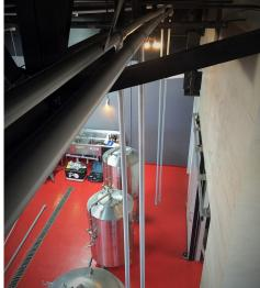
temperatures with ease. It is corrosionresistant, leak-free, maintenance-free, and easily installed. PP-RCT is joined via heat fusion, eliminating the need for glues or solvents. Typically, breweries use 1-inch and 2-inch pipe and fittings. Free Range has
