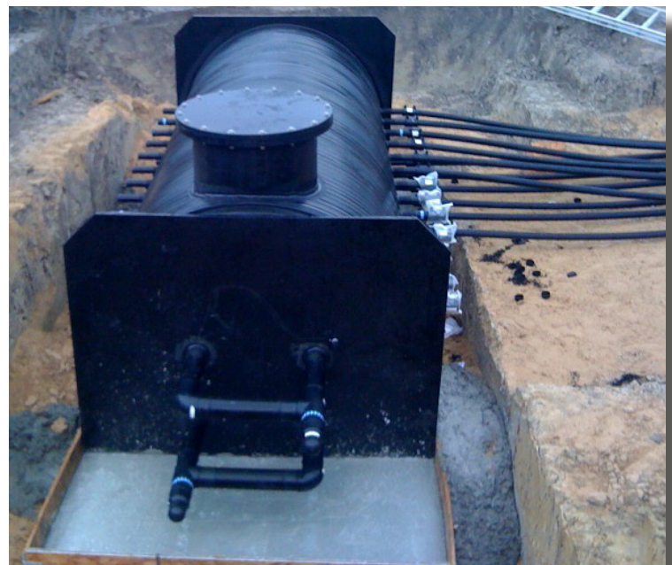
ISCO's custom-fabricated geothermal vault. The installation of the vault is taking place in this photo.
