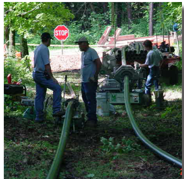
Caveland employees joining HDPE pipe using the butt-fusion method.
