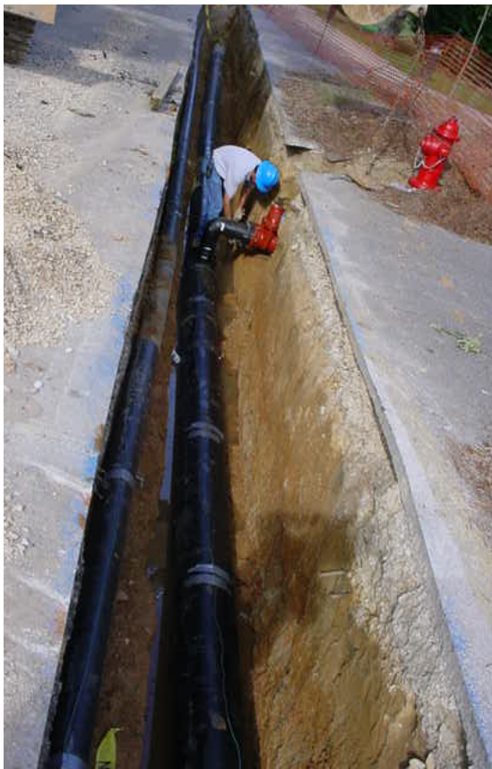
Final installation of a fire hydrant on the large water main next to the 6" main for drinking water.
