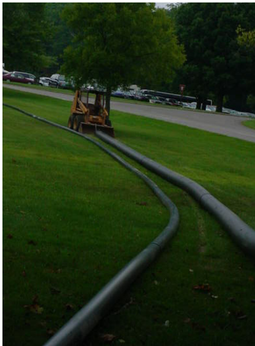
Long runs of HDPE pipe before installation which helped with traffic disruption.
