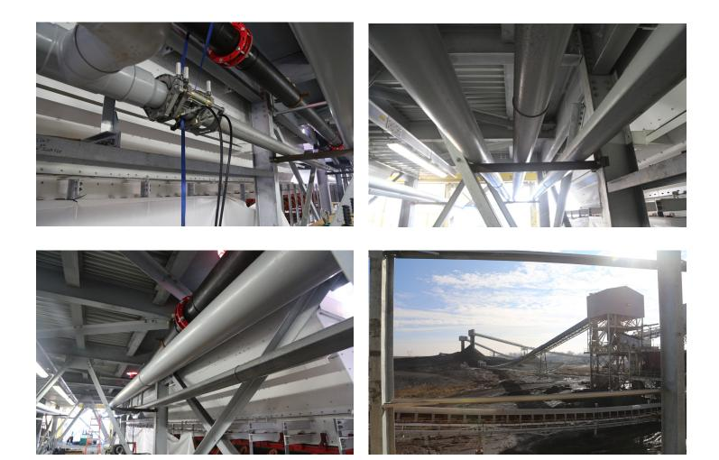
The material is 100% recyclable and environmentally friendly. It lasts significantly longer than traditional pipe materials because it won't corrode. "You don't want to go with steel, of course, especially with slurry," Smith said. "We needed a pipe that would be light enough to hang, but strong enough to handle the pressure. Matt brought PP-RCT to our attention and it sounded like exactly what we needed"
