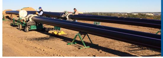
Sliplinging high-density polyethylene makes an aging water line useable again.
