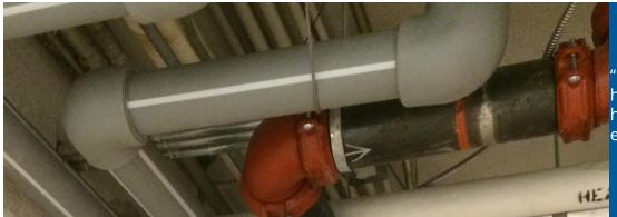
"PP-RCT is connected via heat fusion, a process of heating and joining pipe ends under pressure."
