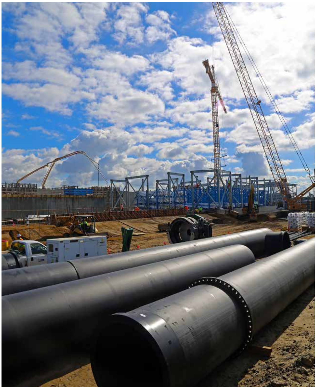
San Diego County Desalination Plant: www.isco-pipe.com/SanDiegoCounty
