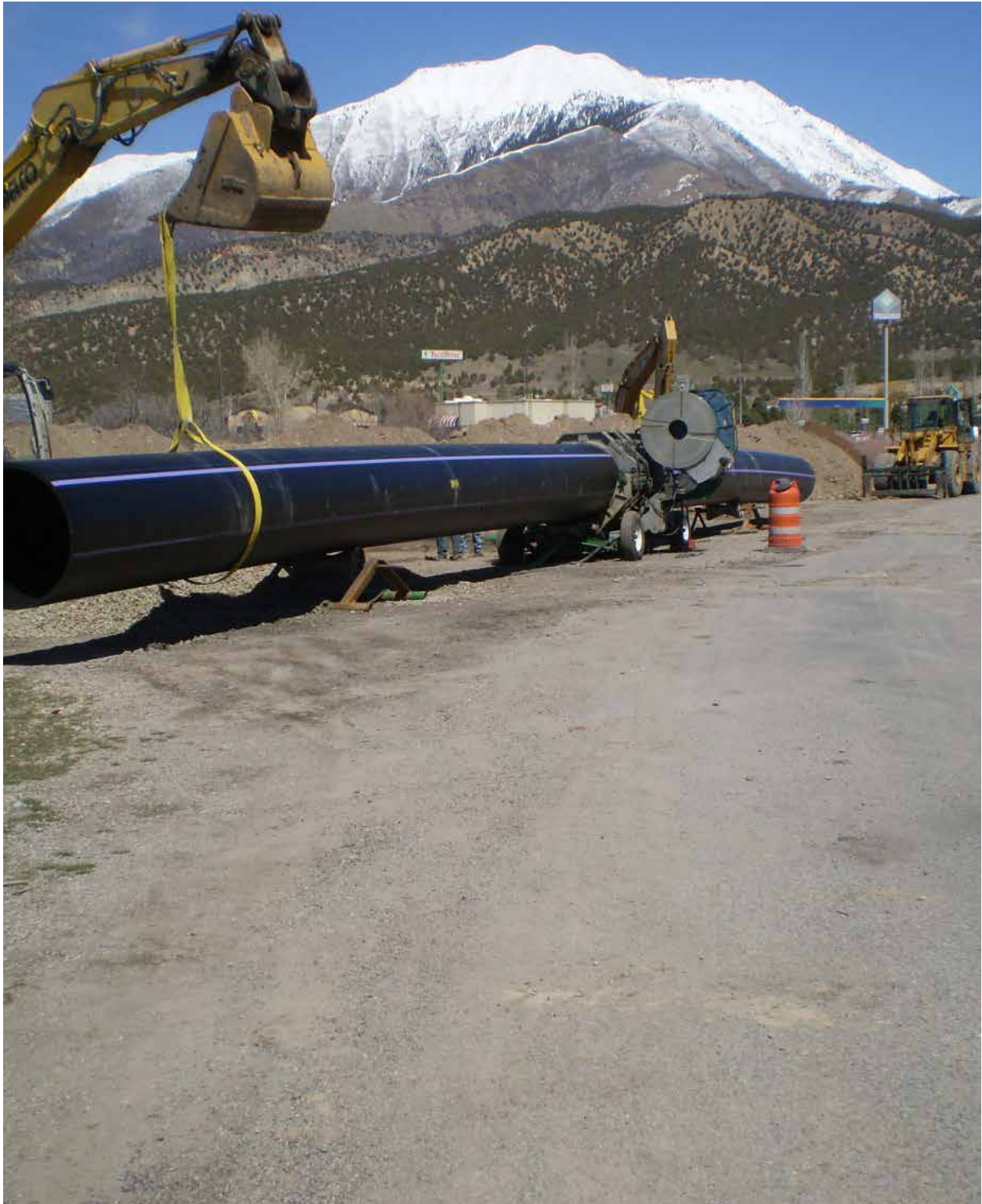
Nephi, Utah - www.isco-pipe.com/CanalUT
