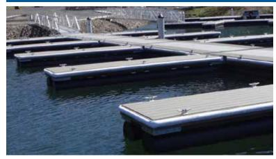
A total of 62 floating docks built for a resort marina in Oregon. 1,160 lineal feet total in 8-,6- and 4-foot-wide combinations. The decking is a composite-style deck made of a wood and plastic combination.
