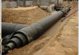
Durable, corrosion-free pipe installed at innovative So. California desalination plant.
